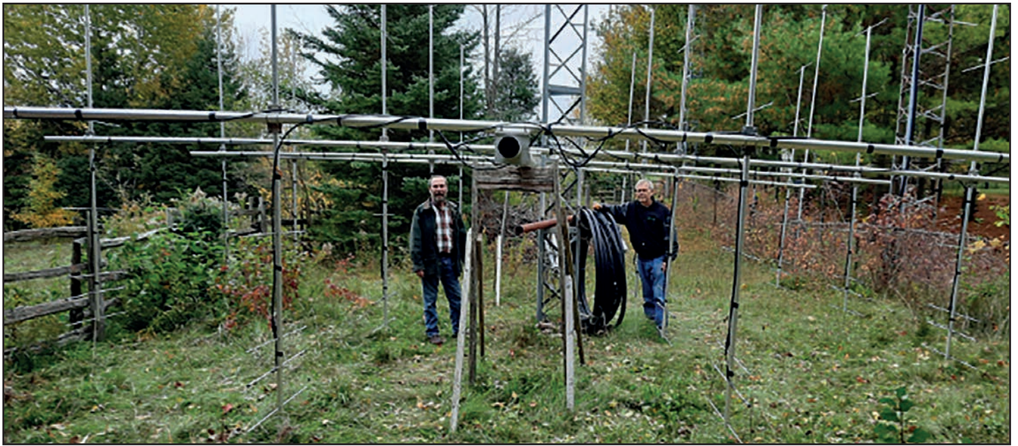
Moonbounce: Bob Morton, VE3WY, shown on the right next to Svend de Bruyn, VE3SWN, has been assembling an array of 16 x 7-element Yagis for 144 MHz EME and plans to get it up on the tower this spring. The array will put FN04 solidly on the EME map, with a KW behind it. Watch for more information in an upcoming issue of The Canadian Amateur magazine.
