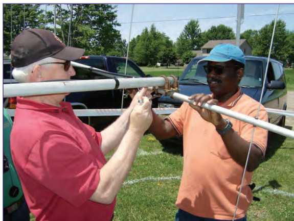
Dick Wilson, VE3WRW (on the left) and Avery Jones, VE3QAP, mount a 2m beam antenna to the top of the mast for the VHF array.
