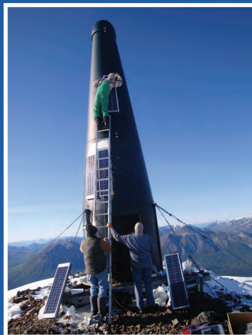
Yukon ARA Solar Panel Upgrade
