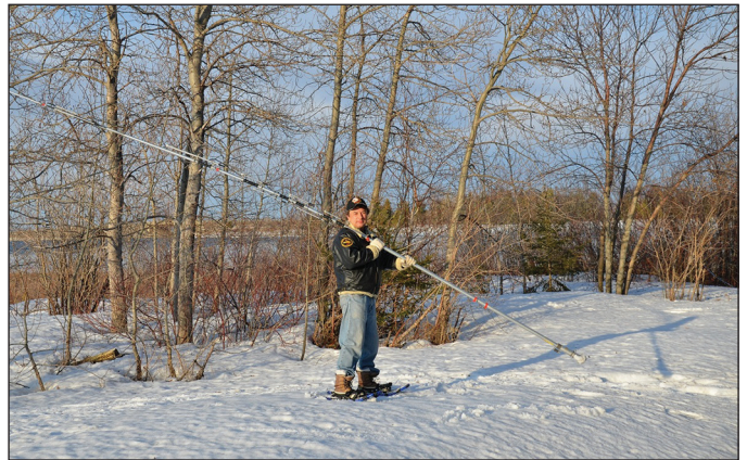
Igor, VE3ZF, installing phasing verticals.
