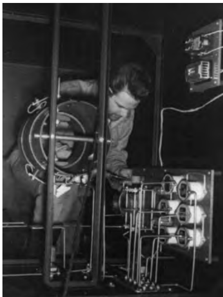
Figure 5: The LF ATU at the base of the Coral Harbour 250-foot tower.
