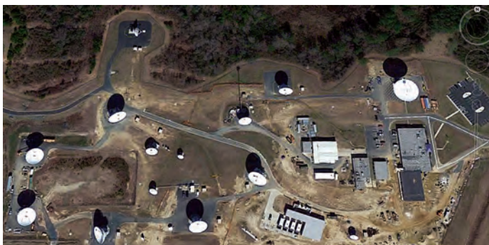
Figure 5: Wallops Island NOAA SCDA Facility (Courtesy Google Earth)
