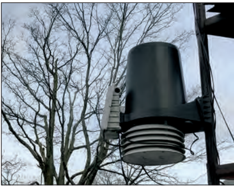
The temperature, humidity and rain gauge module mounted on the tower.
